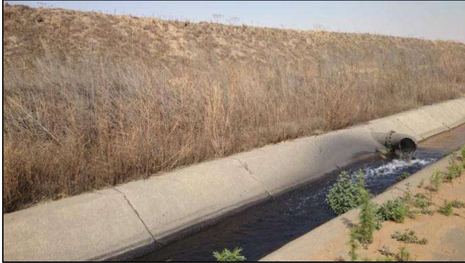
Figure 7-2: Trapezoidal Channel Collecting Water from Discard Dump Penstock Outlets
